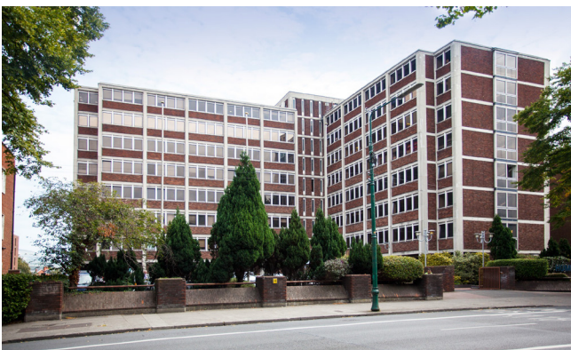
Photo of existing Hume House, Ballsbridge and CGI of approved redevelopment
